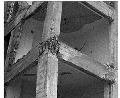
Damaged Beam Columns
