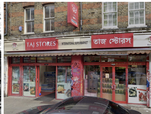
Fig. 41 - Current shopfront of the Taj Stores
