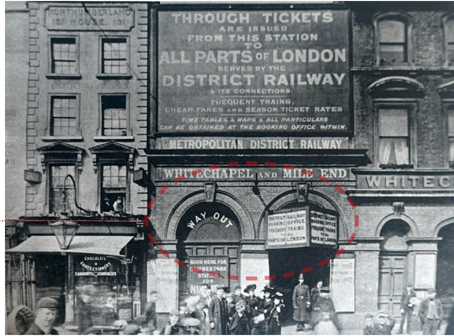
Fig. 46 - Historical picture of Whitechapel Station, dated 1896
