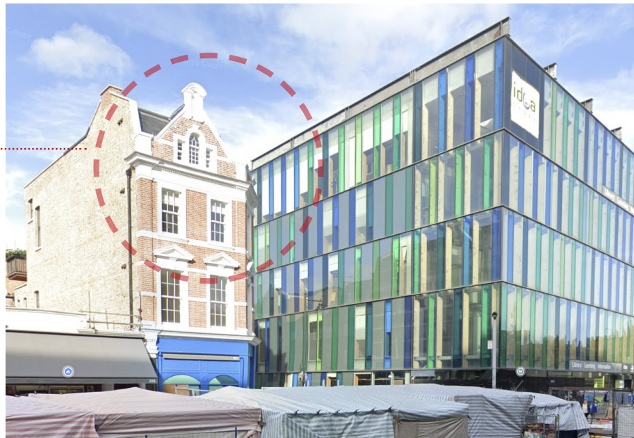
Fig. 45 - Whitechapel Road, turn to Brady Street 2024
