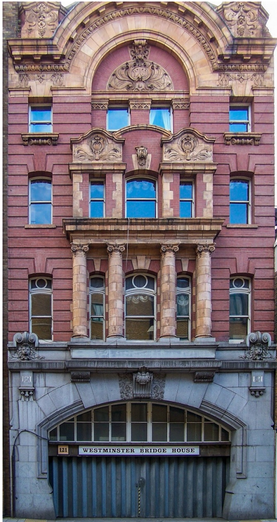
Figure 9 – Westminster Bridge House - the second station for the London Necropolis Railway
