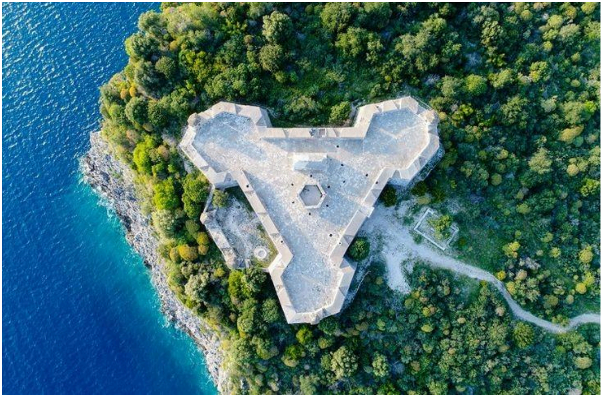
Fig 8 - Aerial view of Porto Palermo Castle
