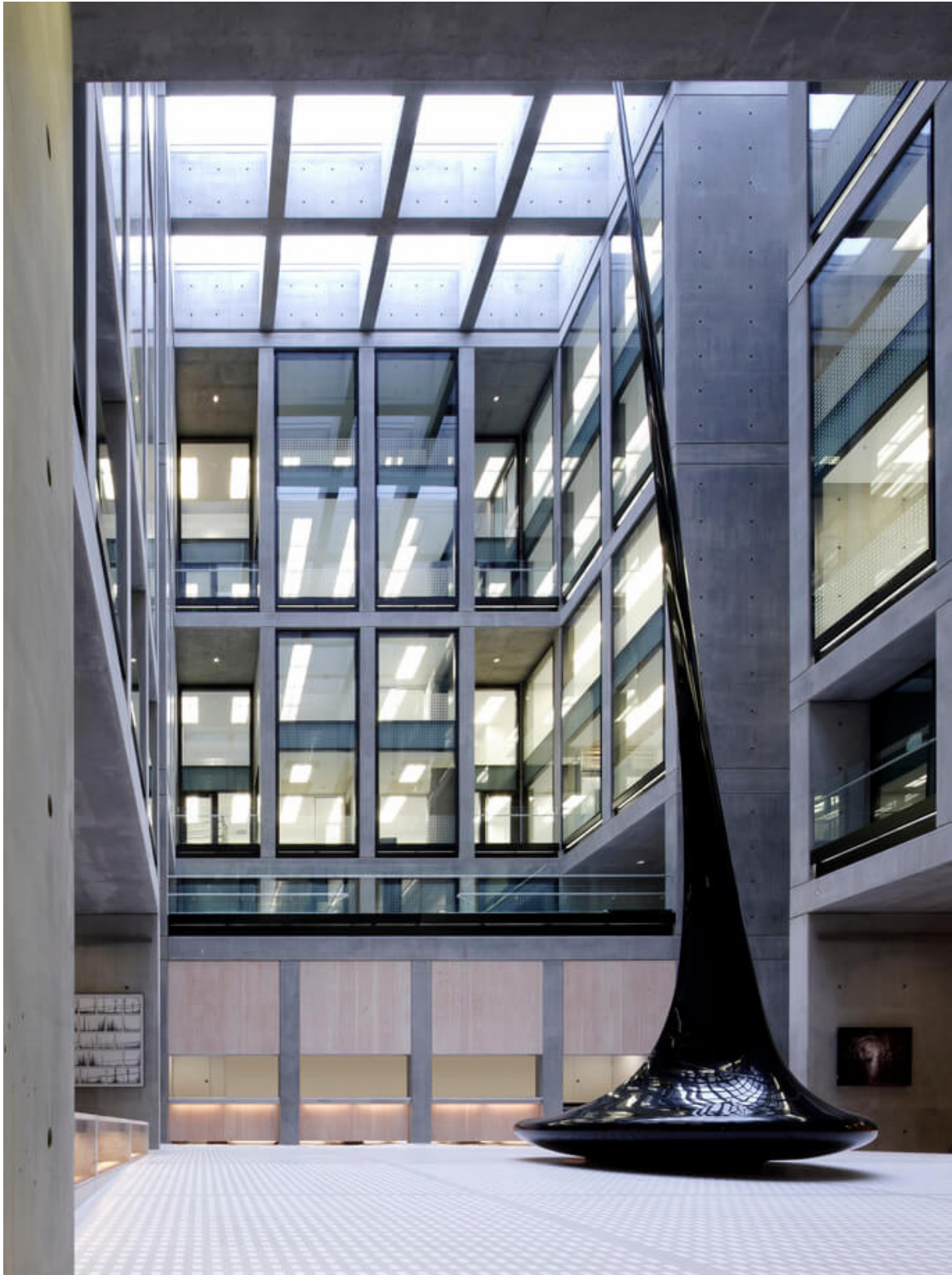
Fig. 5B The completed Angel Building atrium.
