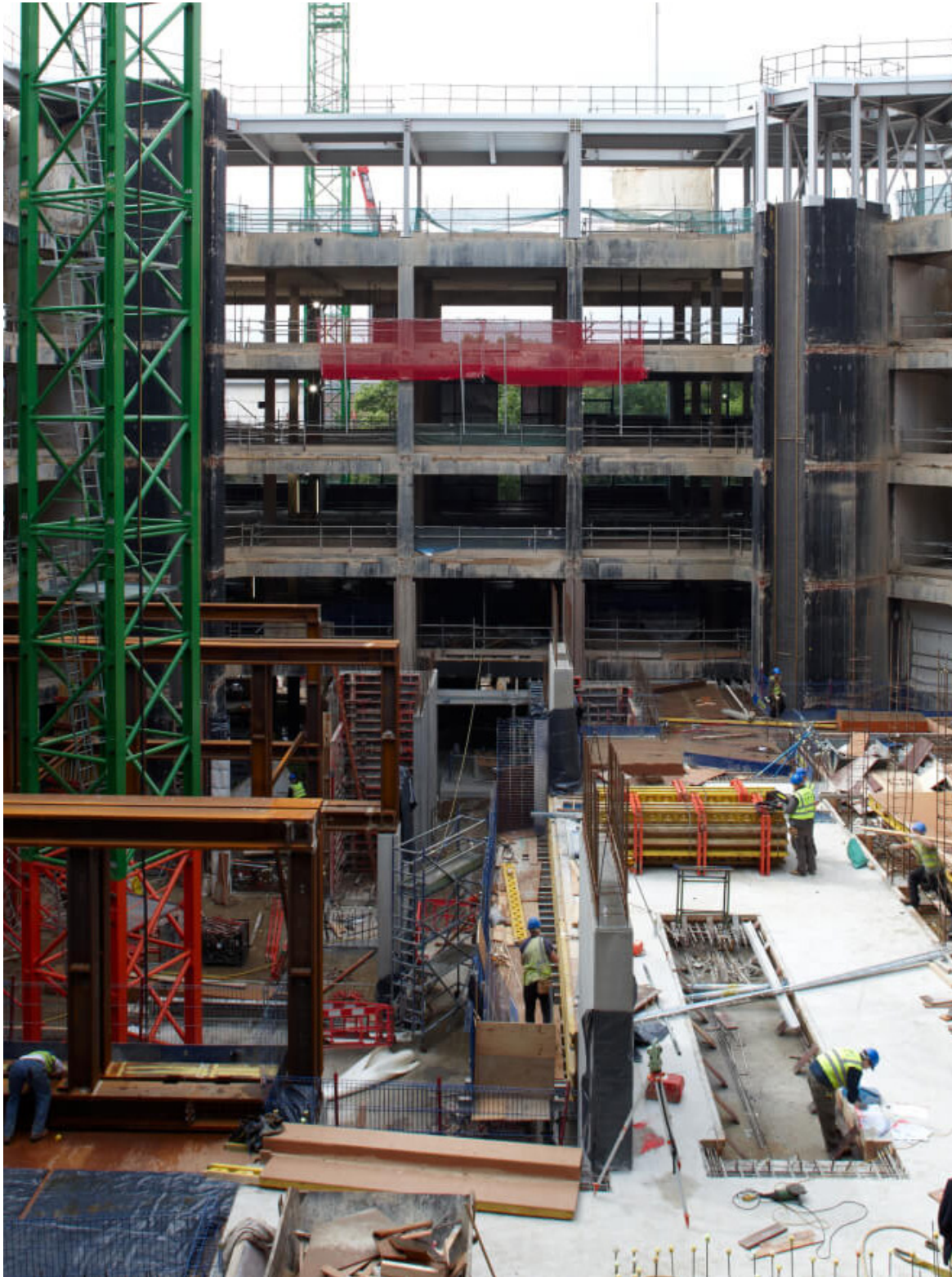
Fig . 5A The Angel Building, Islington, during works.
