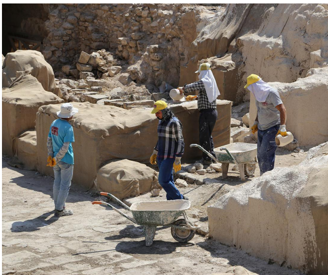
Figure 15: Works on the ruins of the Koç Mosque in 2018 show workers casting a protective layer to prevent the ruins from moving underwater (İLKHA, 2018).
