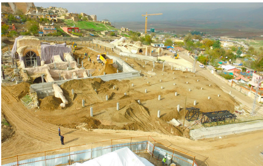
Figures 16: The Koç Mosque and Sultan Süleyman Han Complex were mummified under the same concrete shell. A photograph taken in 2018 shows the various layers applied to the ruins at the old site before they were submerged underwater (Sevgi, 2024, p.65).
