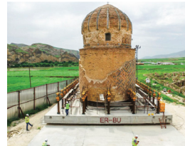
Lifting taking place
