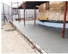
30cm reinforced concrete foundation
