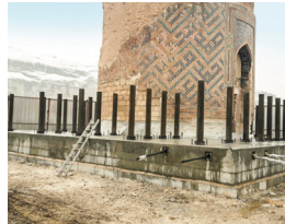
Installing lifting jacks
