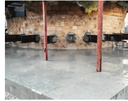
Second layer of foundation
