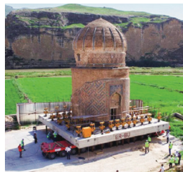
SPMT positioned underneath for relocation
