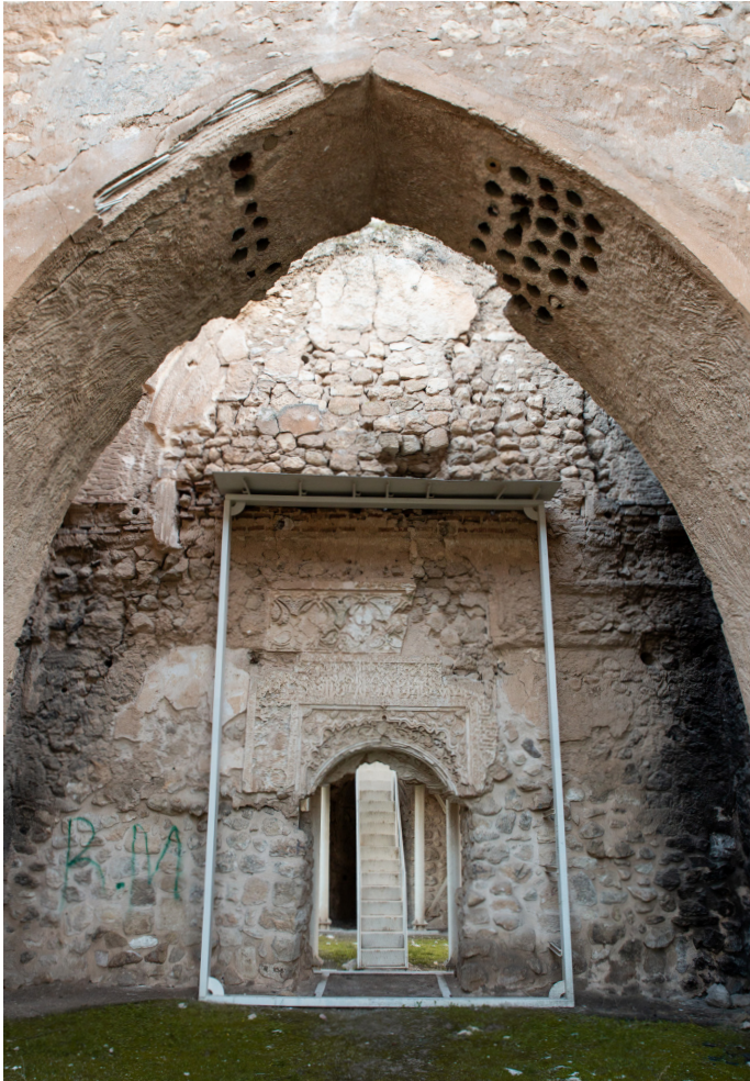
Figure 13: Entrance to the iwan of the Koç Mosque showing the temporary structural supports the load of the building (Little, 2017)
