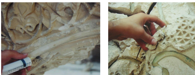
Figures 14: Koç Mosque's iwan facade being repaired and reconstructed during the conservation works in 2000 (Eskici, 2006, p.96)
