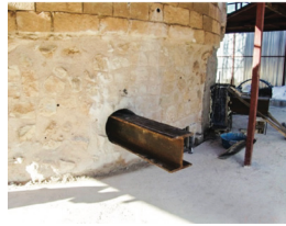
Installing the H-profile steel beams
