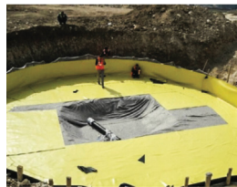
New foundations protection layer
