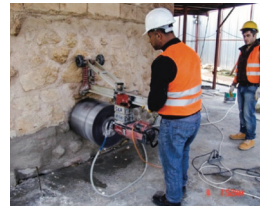
Drilling holes to the lower base
